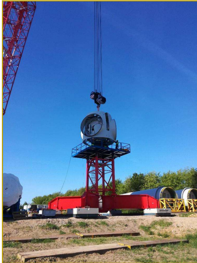
Assembly platform for rotor star
