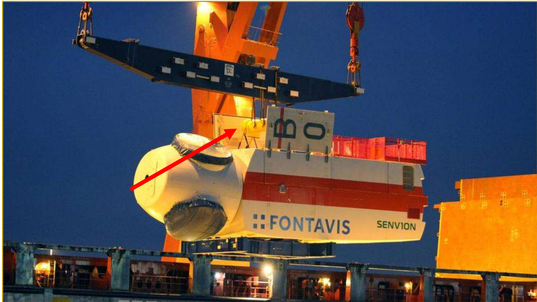
Nacelle lifting beam SWL 480 t – manual centre of gravity adjustment
