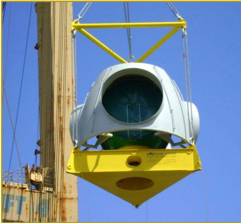
Transport frame and spreader for rotor hub 5 MW
