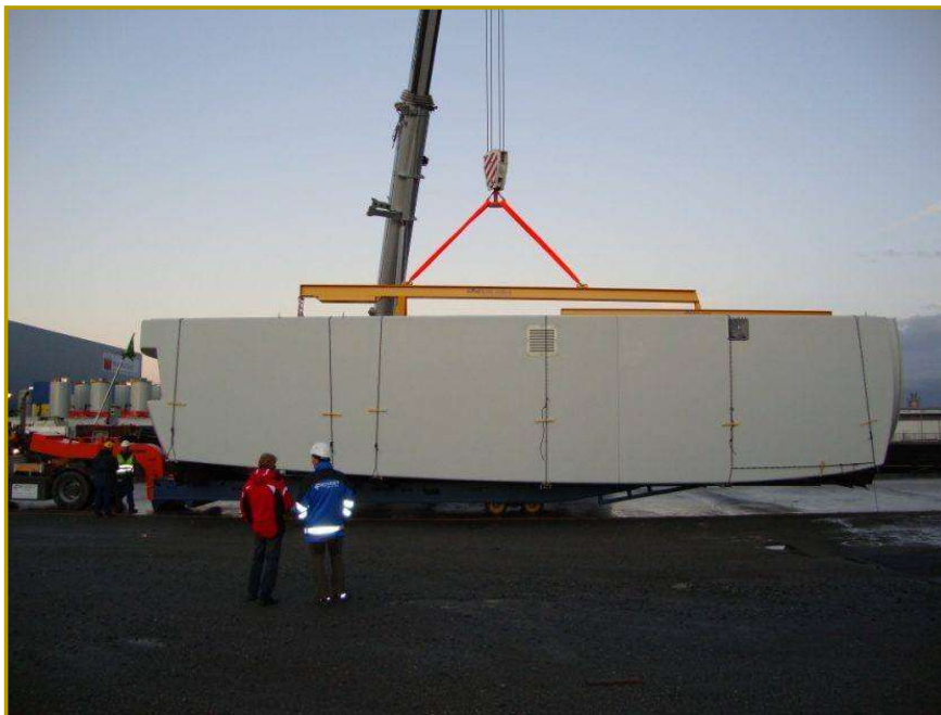
Lifting beam system for nacelle cover 6 MW
