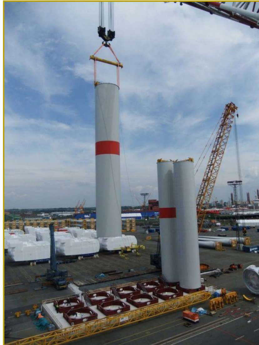
Lifting device, spreader and tower SWL 280 t
