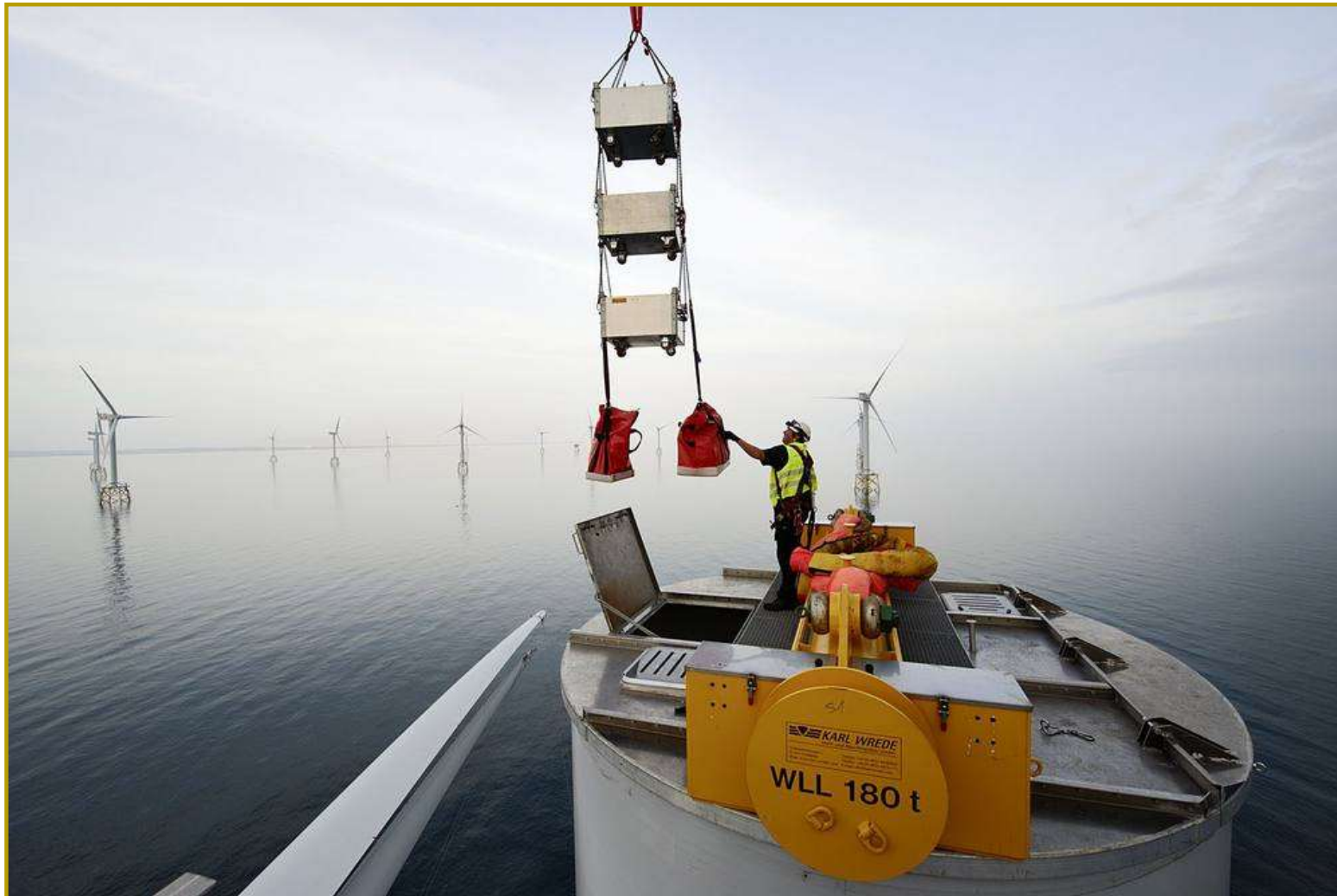
Lifting device for tower SWL 280 t with cover plate
