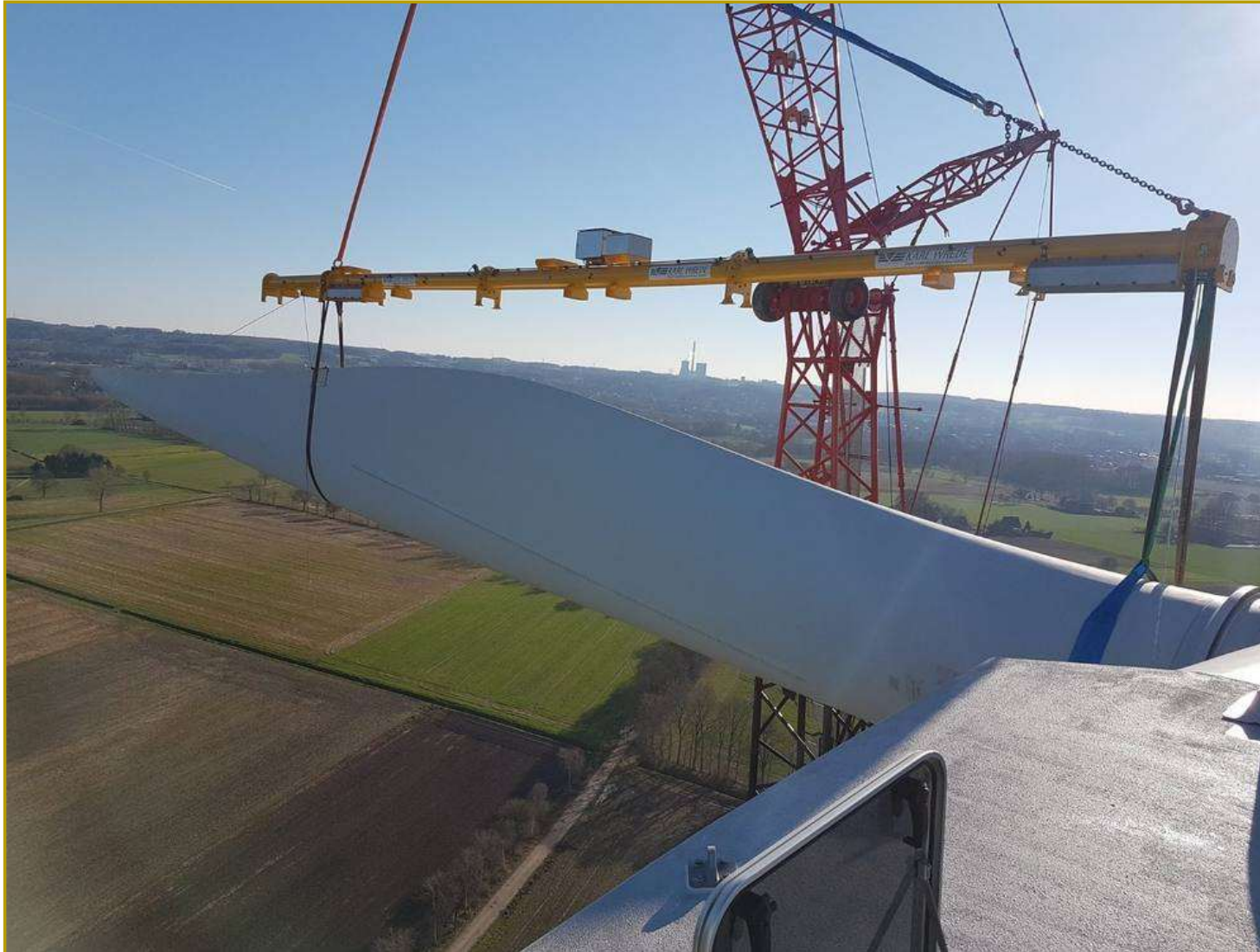
Single blade installation beam
