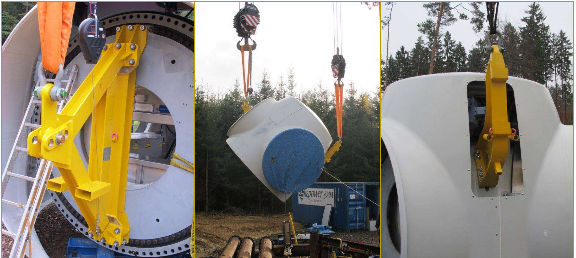
Lifting beam system for lifting and turning the hub 3 MW
