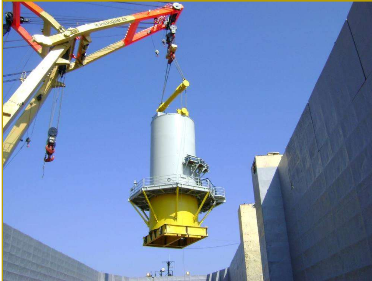
Spreader, lifting beam and transport frame for tower section 5 MW
