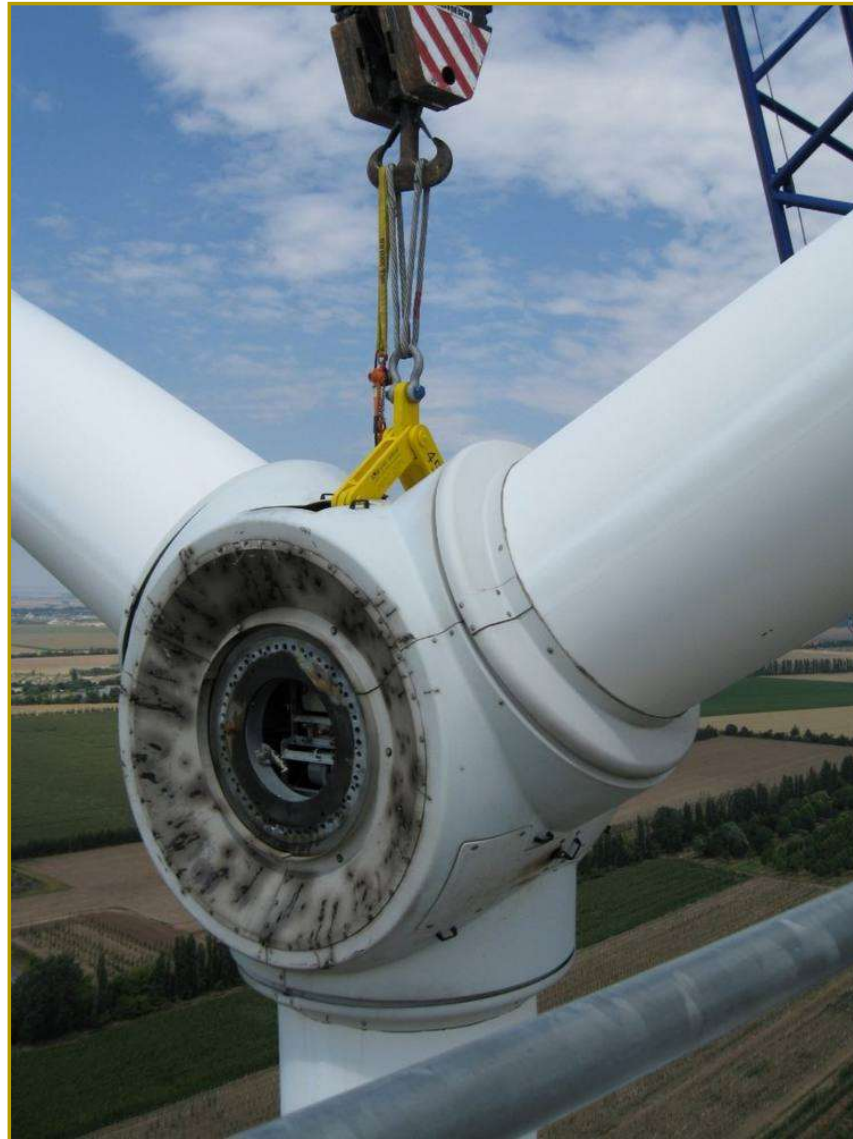
Rotor star lifting beam 2 MW
