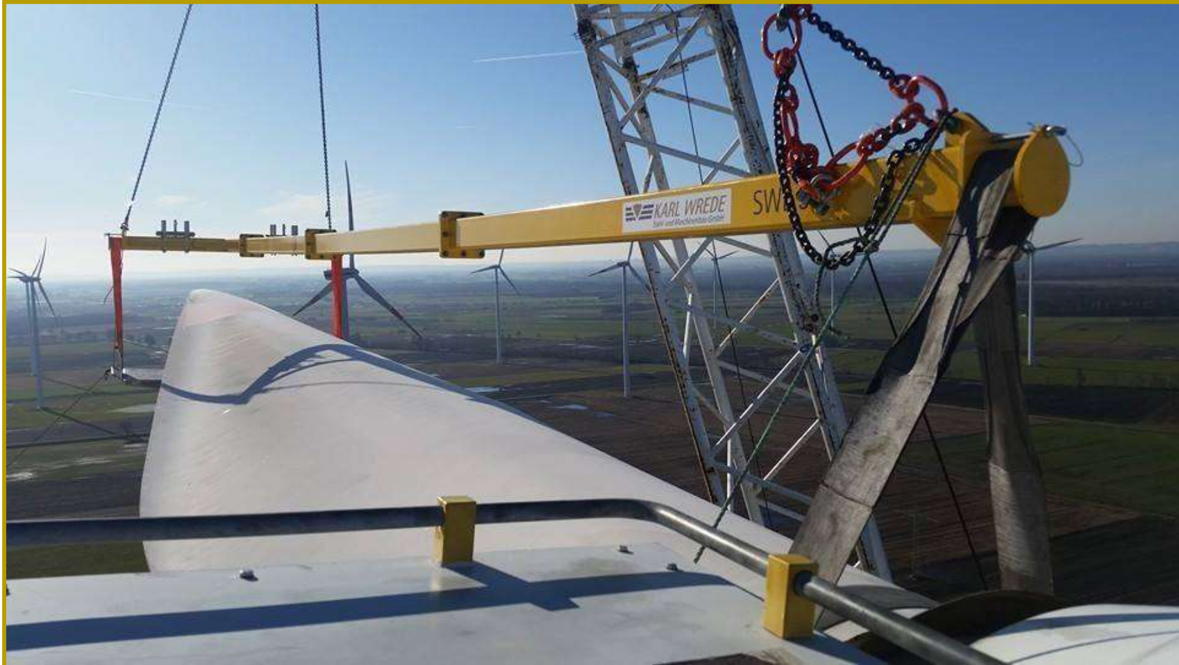
Single blade installation beam
