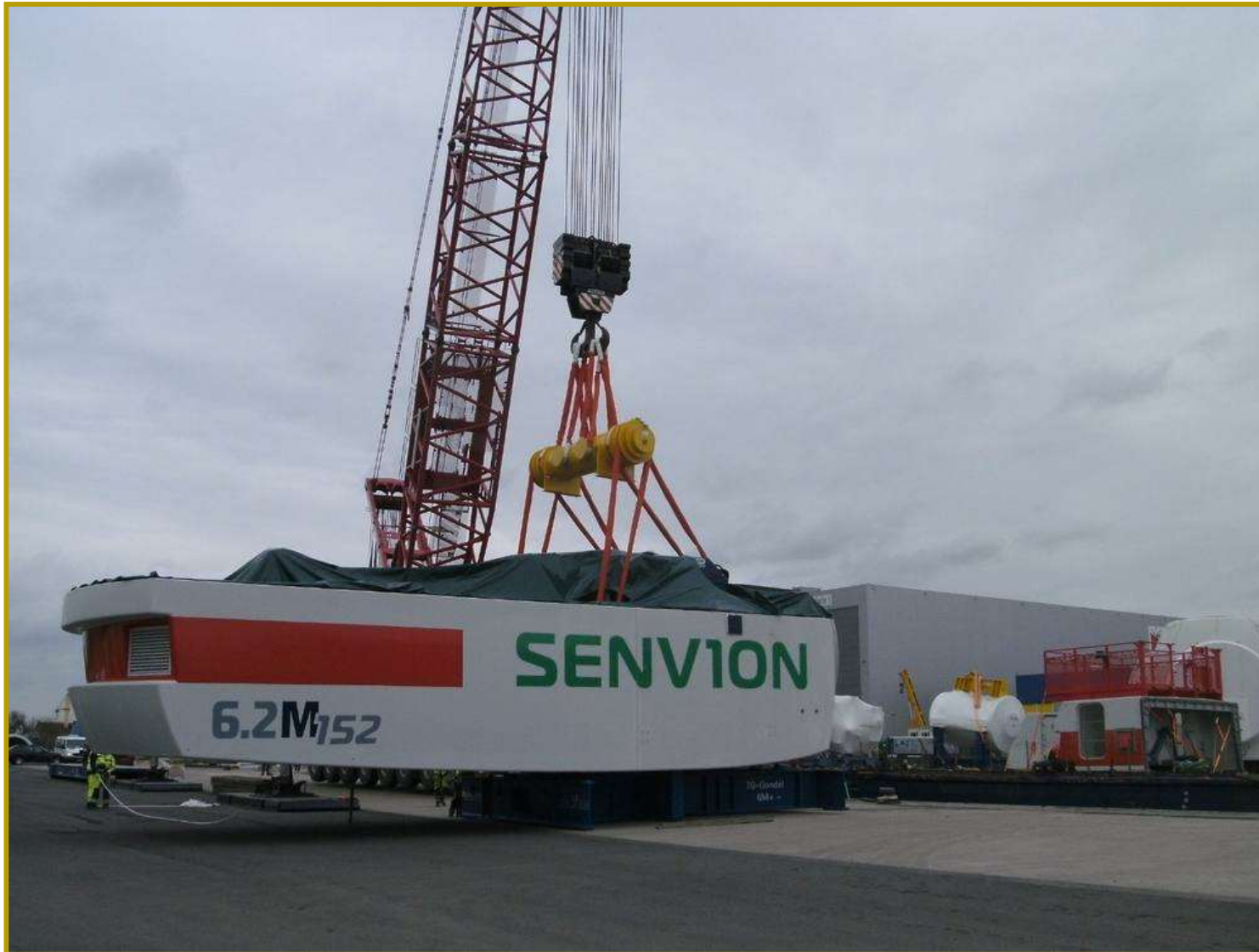
Nacelle lifting beam SWL 480 t
