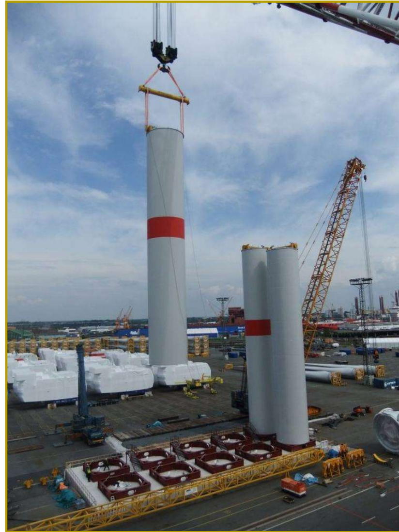
Spreader SWL 280 t and tower lifting device in operation
