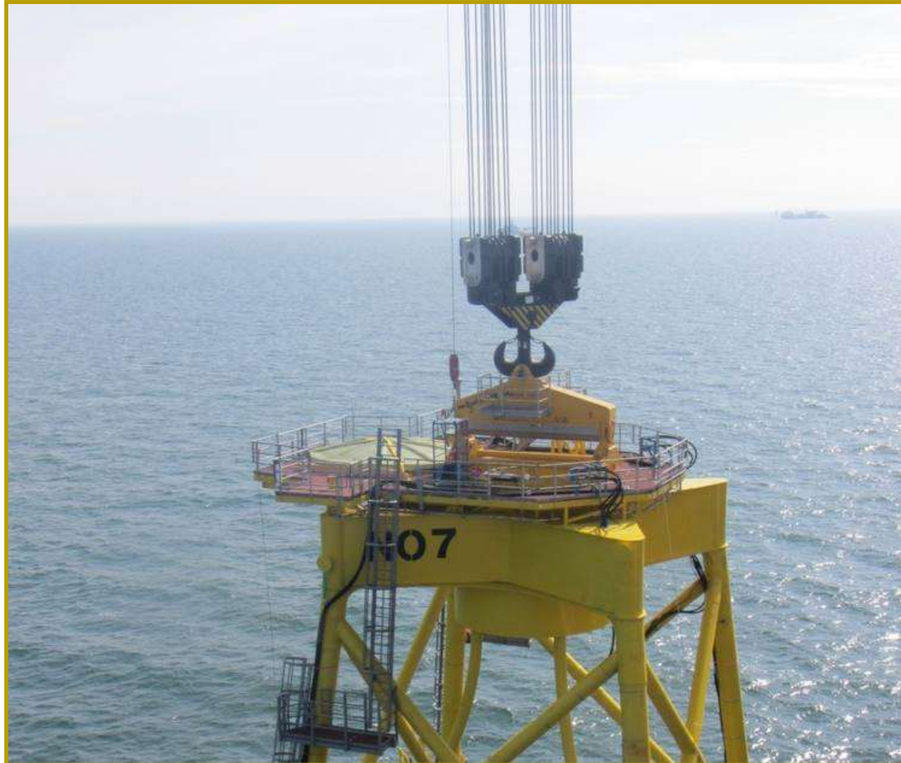
Installation beam SWL 650 t in operation
