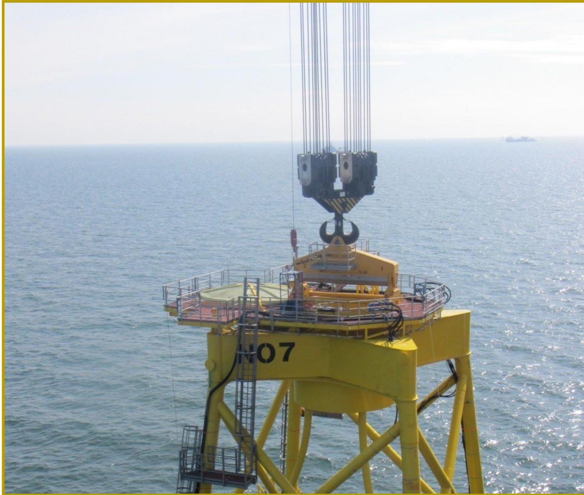
Installation lifting beam - SWL 650 t in operation
