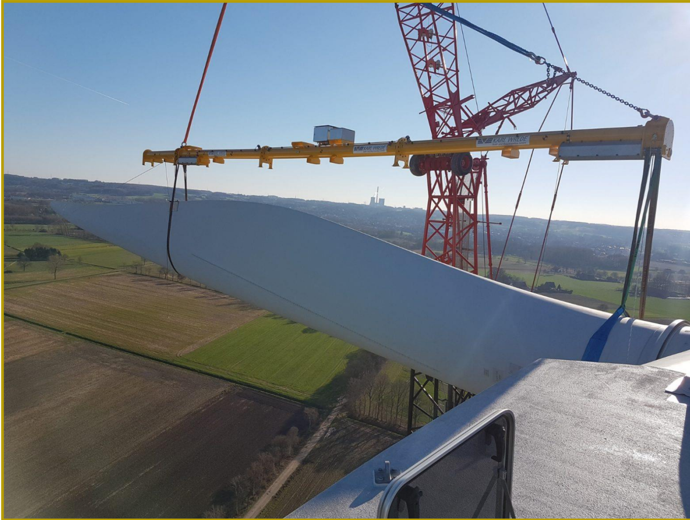
Remote-controlled single-blade installation lifting beam
