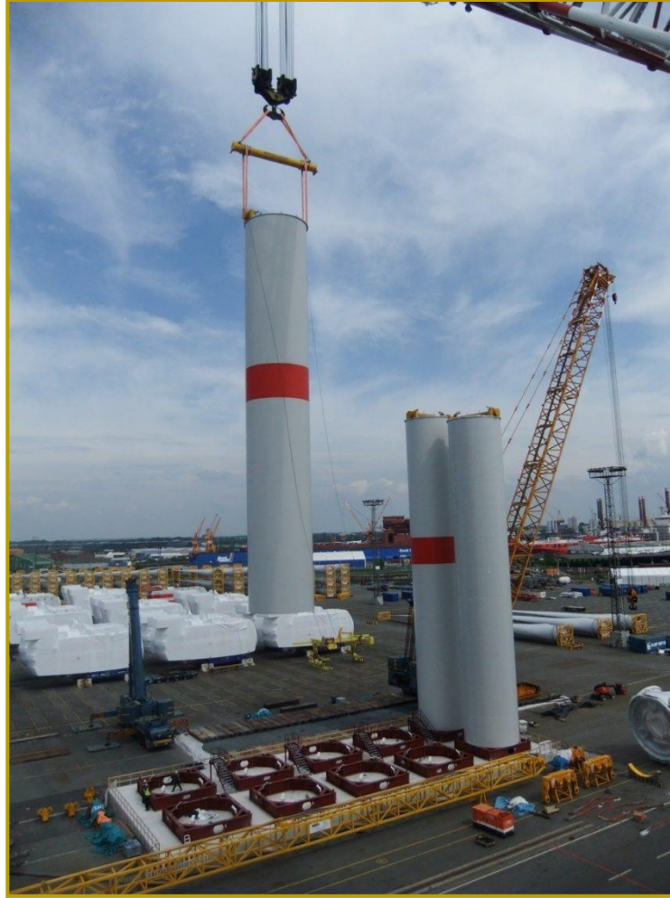
Spreader beam - SWL 280 t and tower lifting device in operation
