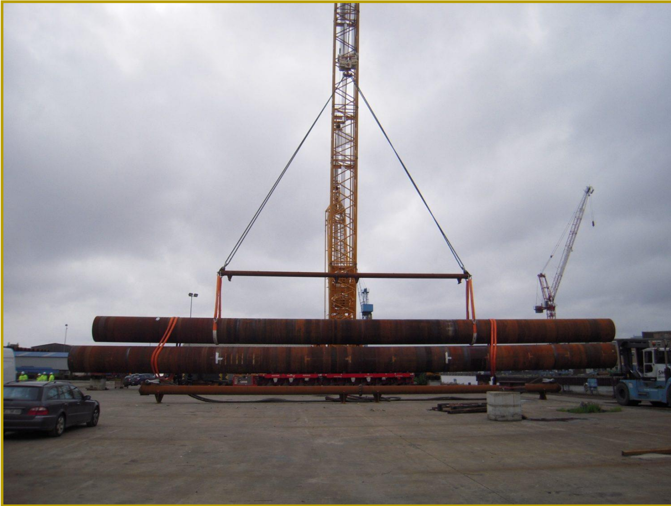
Pile lifting tool - SWL 270 t - l = 25 m
