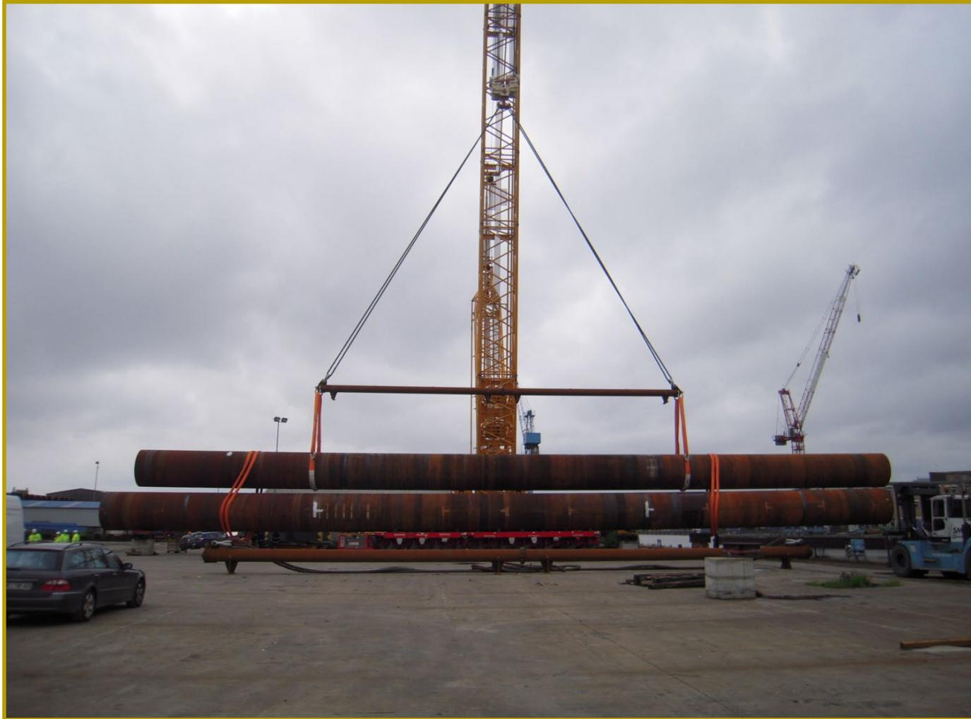
**Pile lifting tool – SWL 270 t – l=25 m**
