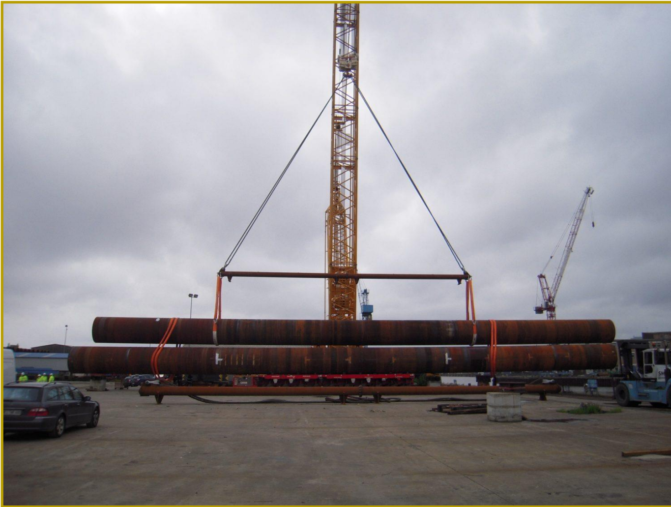
Pile lifting tool – SWL 270 t – l=25 m
